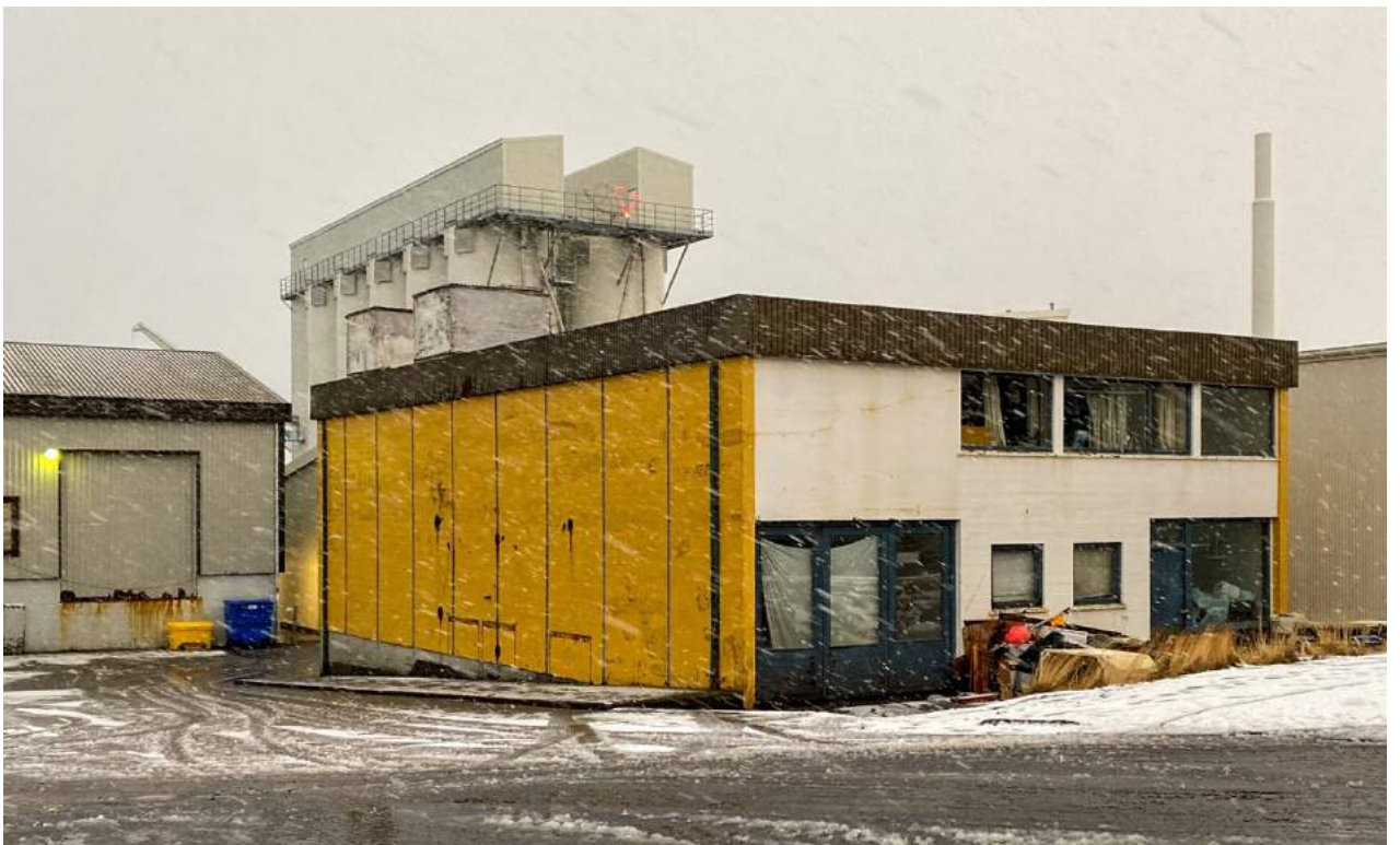
Figure 20: Vopnafjörður power plant (Aðalbjörnsson)
