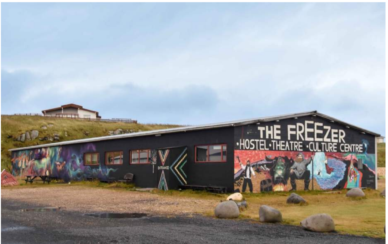
Figure 16: Rif - Freezer Hostel and Culture Centre (Kampfner)
